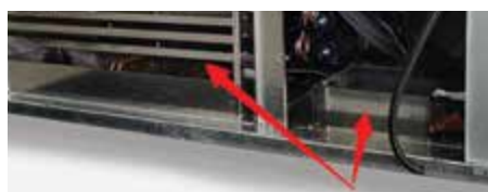
Drain pan heating element for condensation evaporation
