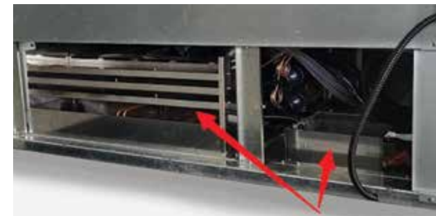
Drain pan heating element for condensation evaporation
