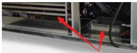
Drain pan heating element for condensation evaporation
